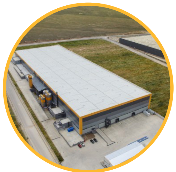
ODE Eskişehir, Turkey Production Facilities
