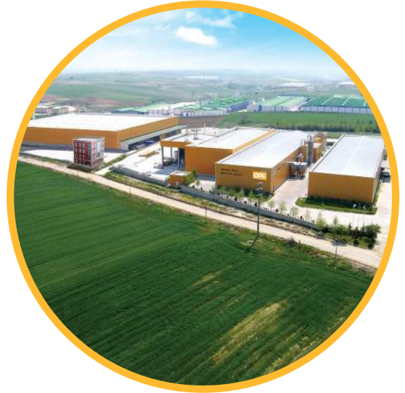
ODE Çorlu/Tekirdağ, Turkey Production Facilities
